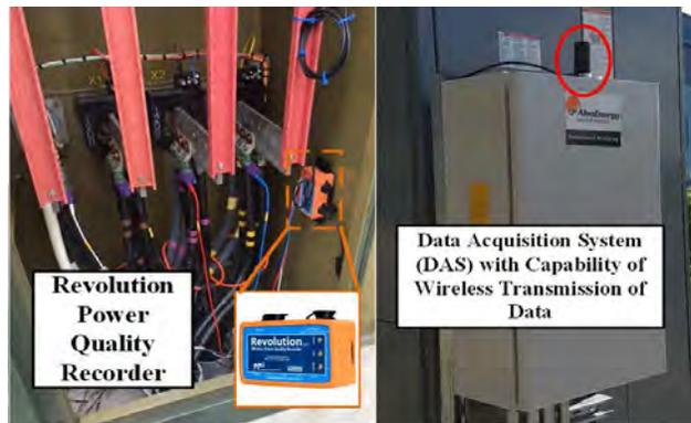
Fig. 2. Revolution Wireless PQ Recorder location (LT sided) and DAS location for measuring time series data from inverters, meter and weather station and securely stores in a cloud server
